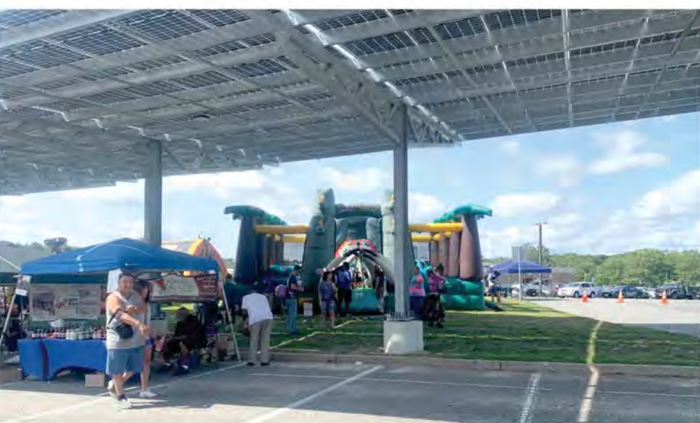
The solar carports, seen here on Pirate's Day at Russell O. Brackman Middle School, provide shelter alongside their environmental benefits. (Veronica Flesher/Patch)
